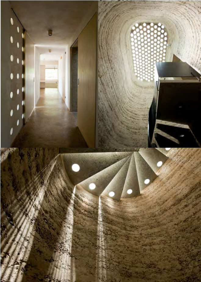
Rammed earth house, Rauch family home Schlins, Autriche. Martin Rauch, Roger Boltshauser © Beat Bühler
